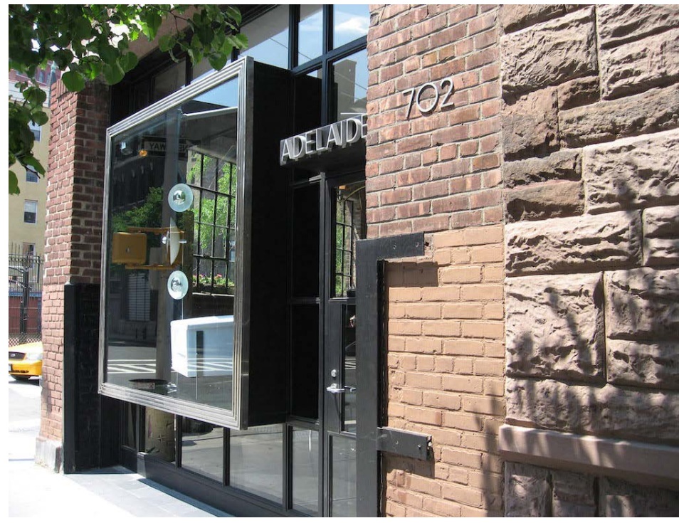
702 Greenwich Street - Greenwich Village His. District Ext. Metal storefront system
