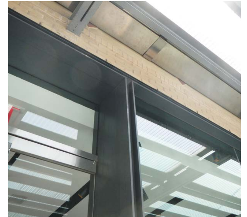
401 West 14th Street - Gansevoort Market Historic District Detail at frame reveal
