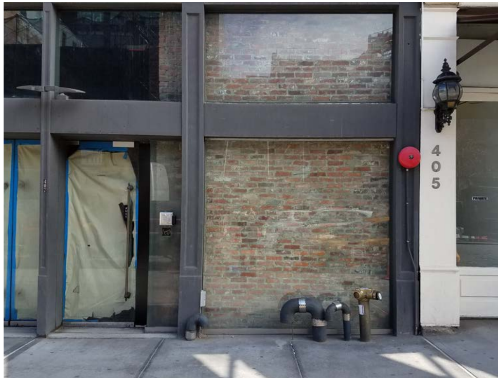
407 West 14th Street - Gansevoort Market Historic District Metal storefront system over existing brick masonry
