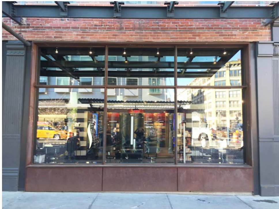
27 Ninth Avenue - Gansevoort Market Historic District Steel storefront system
